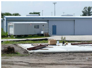
Foundation for new T-hangars
